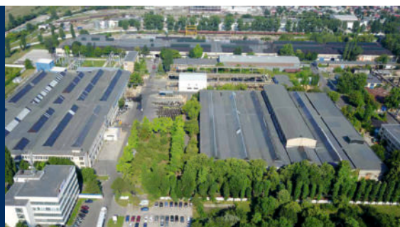
Telecommunication & Data Cables
